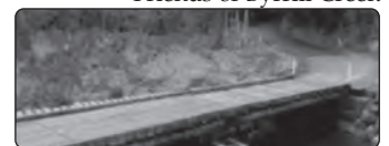
Temporary timber bridge
