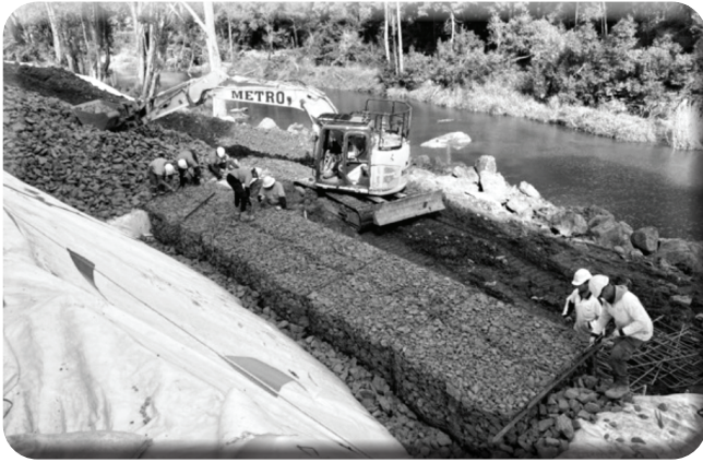
Gabion baskets provide reinforcement
