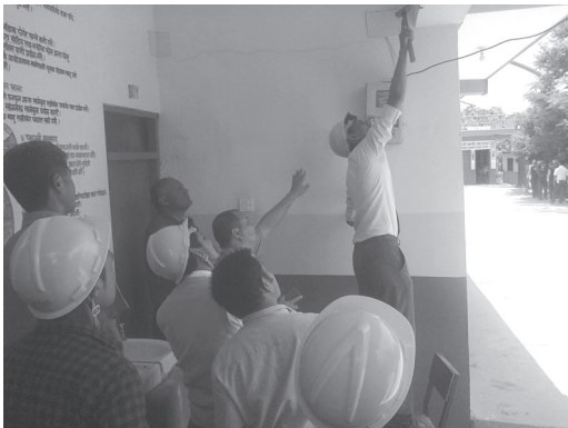
Engineers inspect a cracked wall, above.
